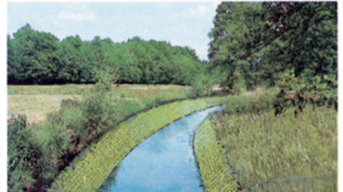
Embankment stabilization.
